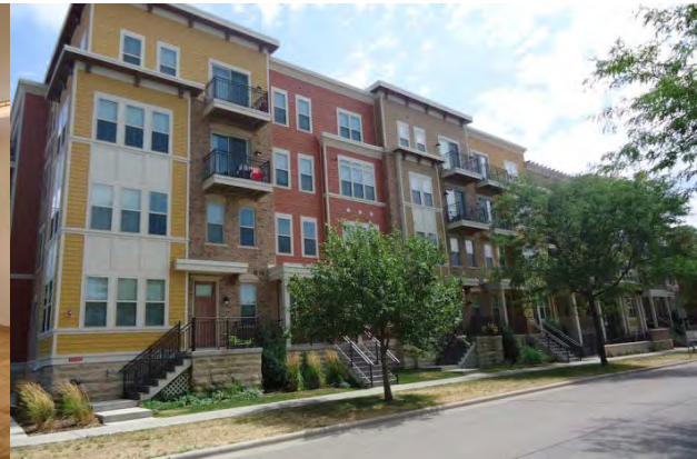
Exterior view from Wilson.
